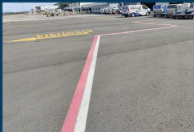
Equipment Clearance Line – vehicles that are parked behind here are clear of aircraft
